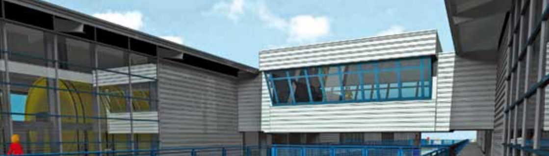
Control station between the eastern pylons
